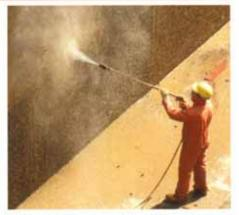
TURBO BLASTER - a jet nozzle combining impact and spray jet - removes dirt and paint quickly and effectively.
