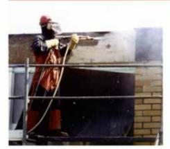
OERTZEN TORNADO - a wide range whirl sandblaster with high surface cleaning power and soft surface treatment.
